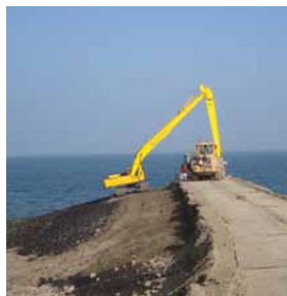
Testing ground for trials with KLEIBERIT Lithobond 579.9
